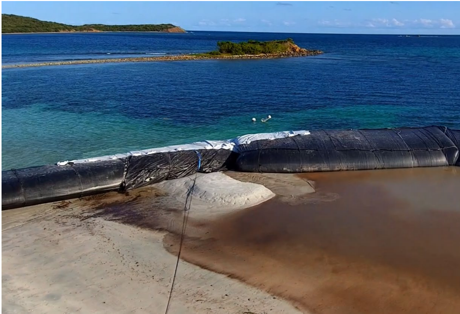
WING - BEACH (east) tube leak
