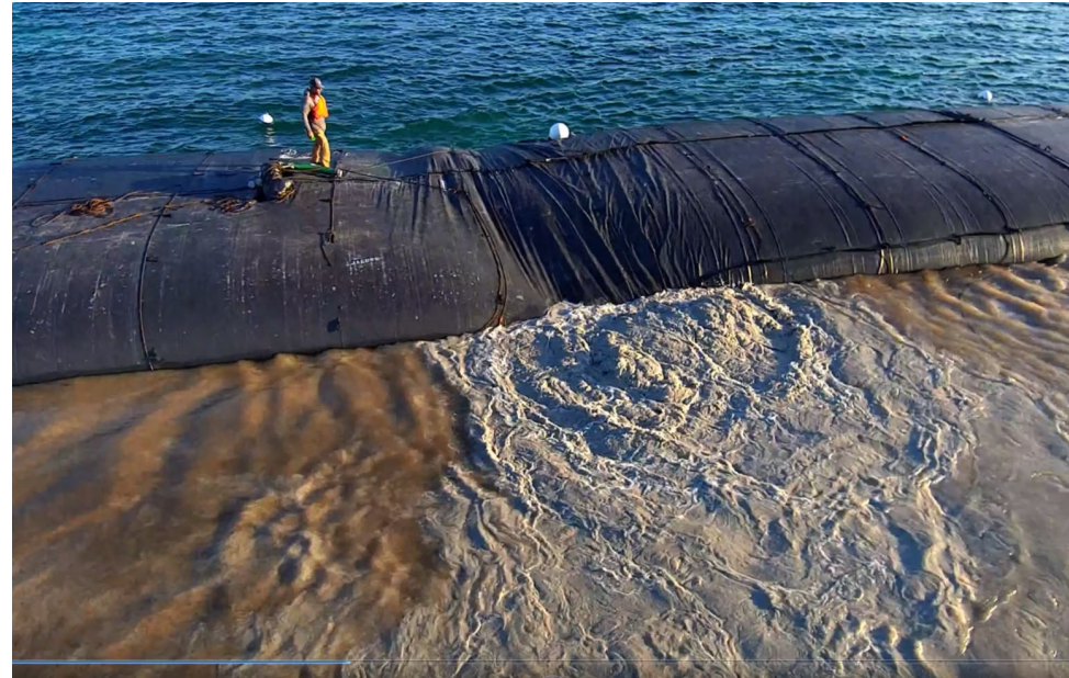
STARTER- WING (west) tube leak
