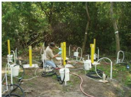
Solutions-IES implementing a remediation pilot test using EOS
